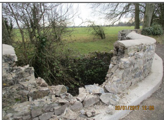
Traffic impact damage 2014 and 2017
