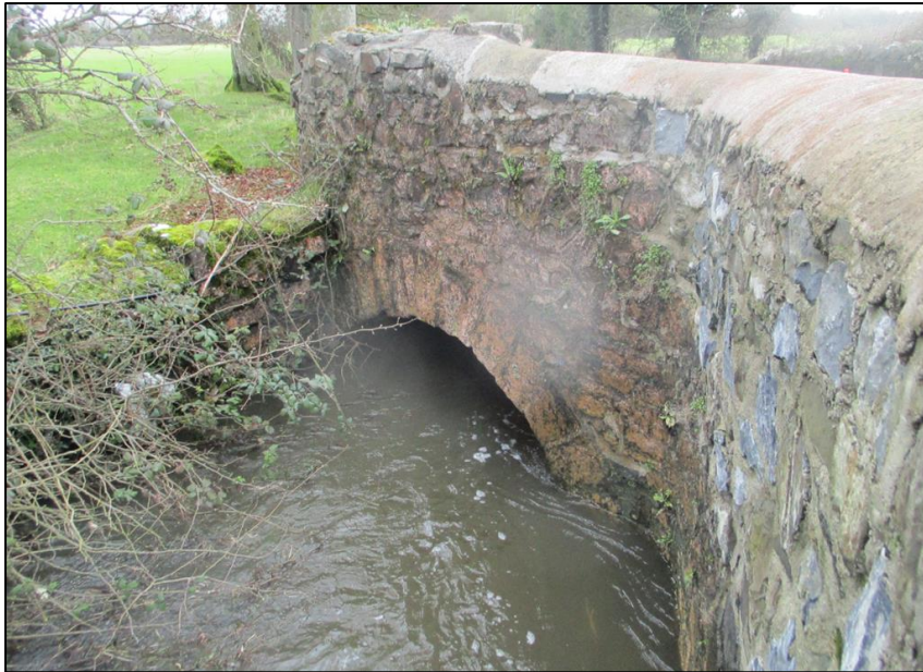
WEST ARCH 2 E face
