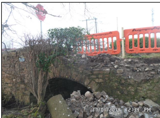
Traffic impact damage 2014 and 2017
